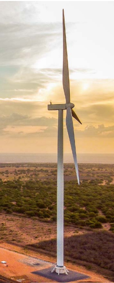
The VSM 3 wind power plant built by Voltalia in the state of Rio Grande do Norte in Brazil.
